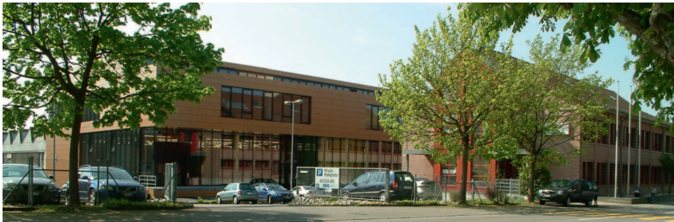
Production plant and administration building of ALESA Ltd
